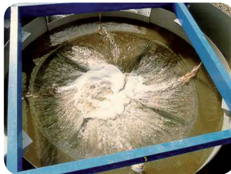
Dynamic backwashing system in operation.
