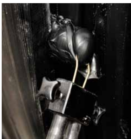
Fig. 4.5.4 Visible sign of welding completion
