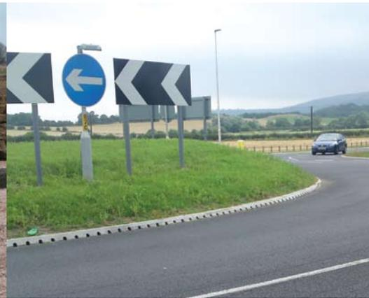
The Lightweight Envirokerb Range of products conform to Manual Handling Regulations, cutting out the cost of any mechanical handling equipment. Installation time is exceptionally quick on the whole Envirokerb System, as well as reducing the RISK of personal injury.
