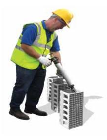
**4** Place Envirodeck unit on the prepared mortar bed using a rubber hammer for adjustment to line and level.
