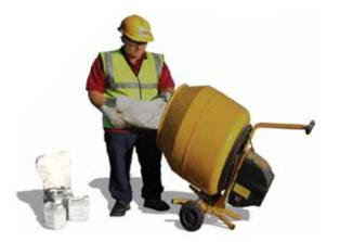
**1.** Envirodeck bedding mortar is mixed in accordance with the recommendations and trowelled to an approx line and level.
