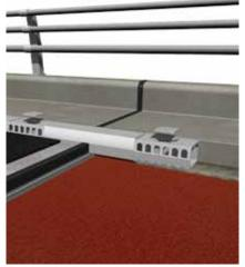
**3** Envirodeck sealant is applied around the end of the unit prior to placement.
