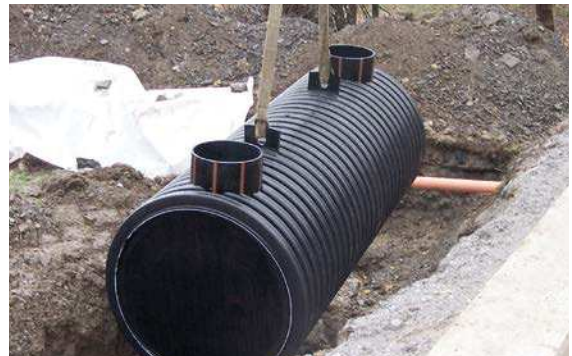
Lowering the sedimentation section into the pipe trenches
