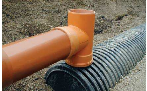
Connecting pipes to the rotatable inlet socket
