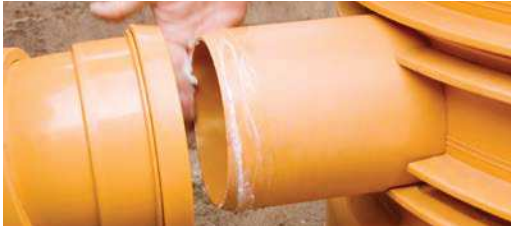
Coating with lubricant
