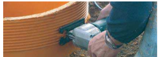
Trimming the chamber cone
