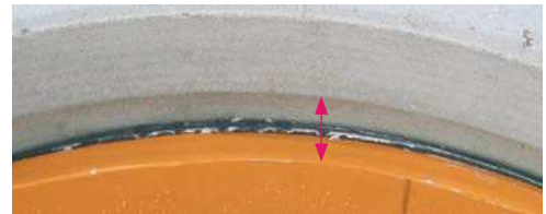
Distance between the cone and the concrete bearing ring
