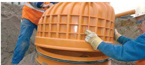
Attaching the cone
