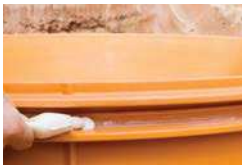
Coating with lubricant
