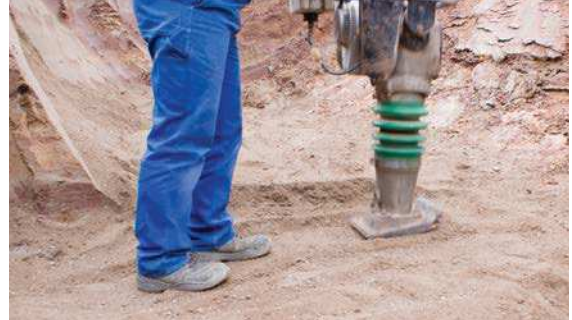
Making the chamber bedding
