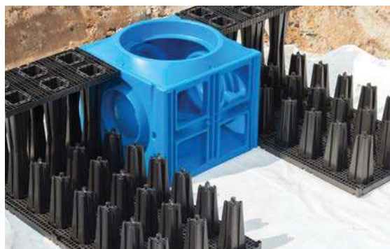
First stages of gravel trench construction with a cleaning channel in the wall structure
