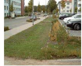
Percolation ditch of a ditch-gravel trench after completion
