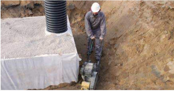
Compacting the work area
