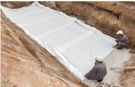
Excavation pit with laid-out geotextile channel
