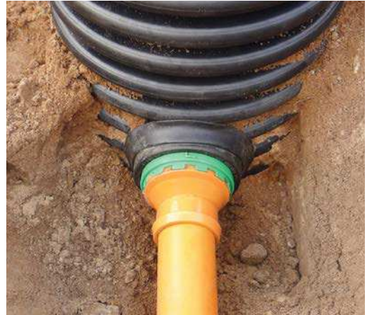
Connecting the ventilation to the chamber extension using AWADOCK
