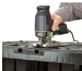
Cutting the base element along the cutting guide
