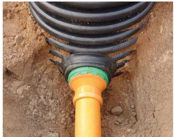
Connecting the ventilation to the chamber extension using AWADOCK
