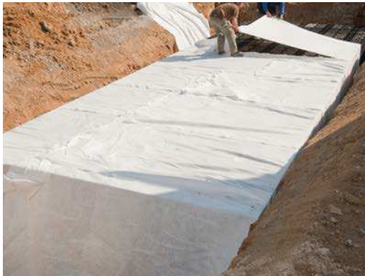
RAUSIKKO Box gravel trench with RAUMAT geotextile filter
