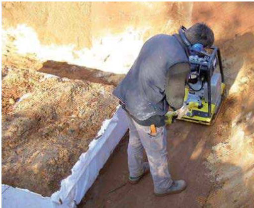
Compacting the work area
