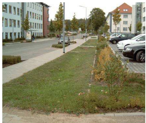
Percolation ditch of a completed ditch-gravel trench
