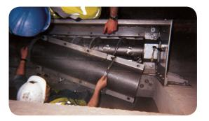
The internal components of the Heliscreen are mounted on the 'wet' (sewer) side of the weir. The main components are easily accessible from the 'dry' side for maintenance or inspection.
