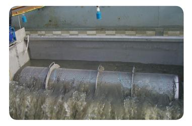
Flows enter the chamber causing water levels to rise, initiating the rotation of the helical brush mechanism on the influent side of the screen, and begins to flow through the Heliscreen®'s semicylindrical stainless steel perforated screen (red arrow).
